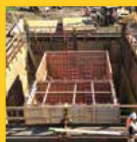
Two bay sheeted pit—re-braced
