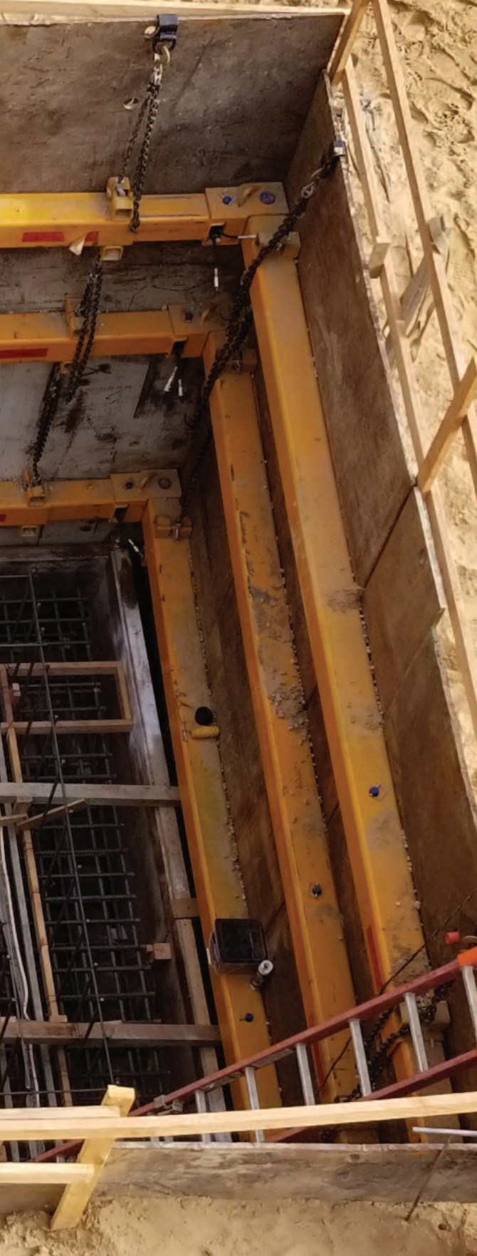
AEX Aluminum Framed Shield
