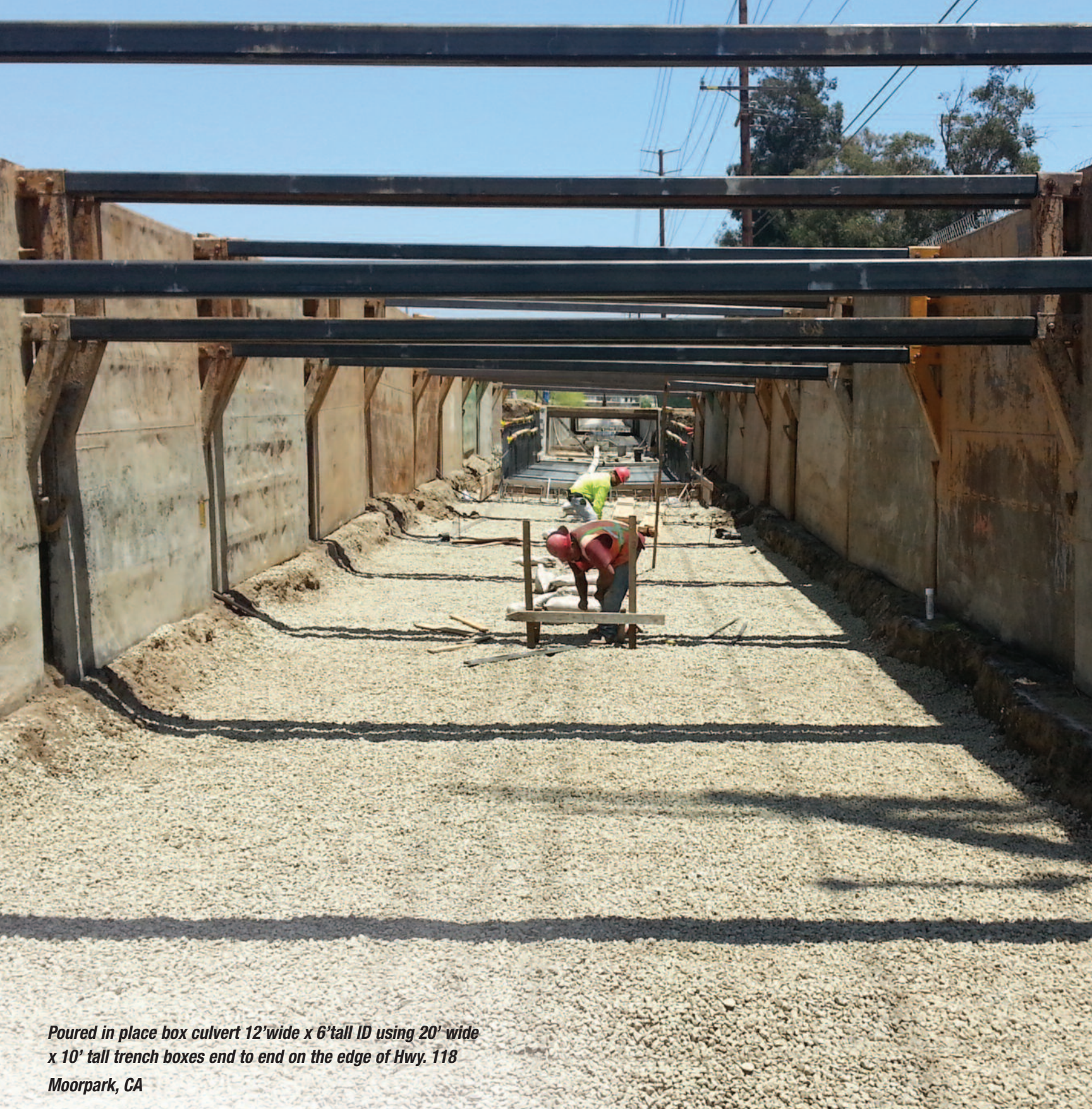
Flex Shield™ Trench Box
