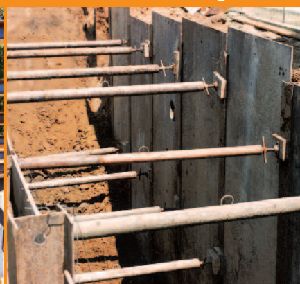
Screw Jacks & Shoring Plates
