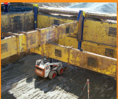
Slide Rail Extended 4-Sided Pit
