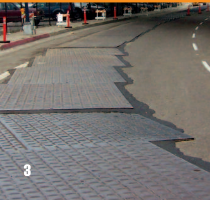
Trench Tops™ (Steel Plates)
