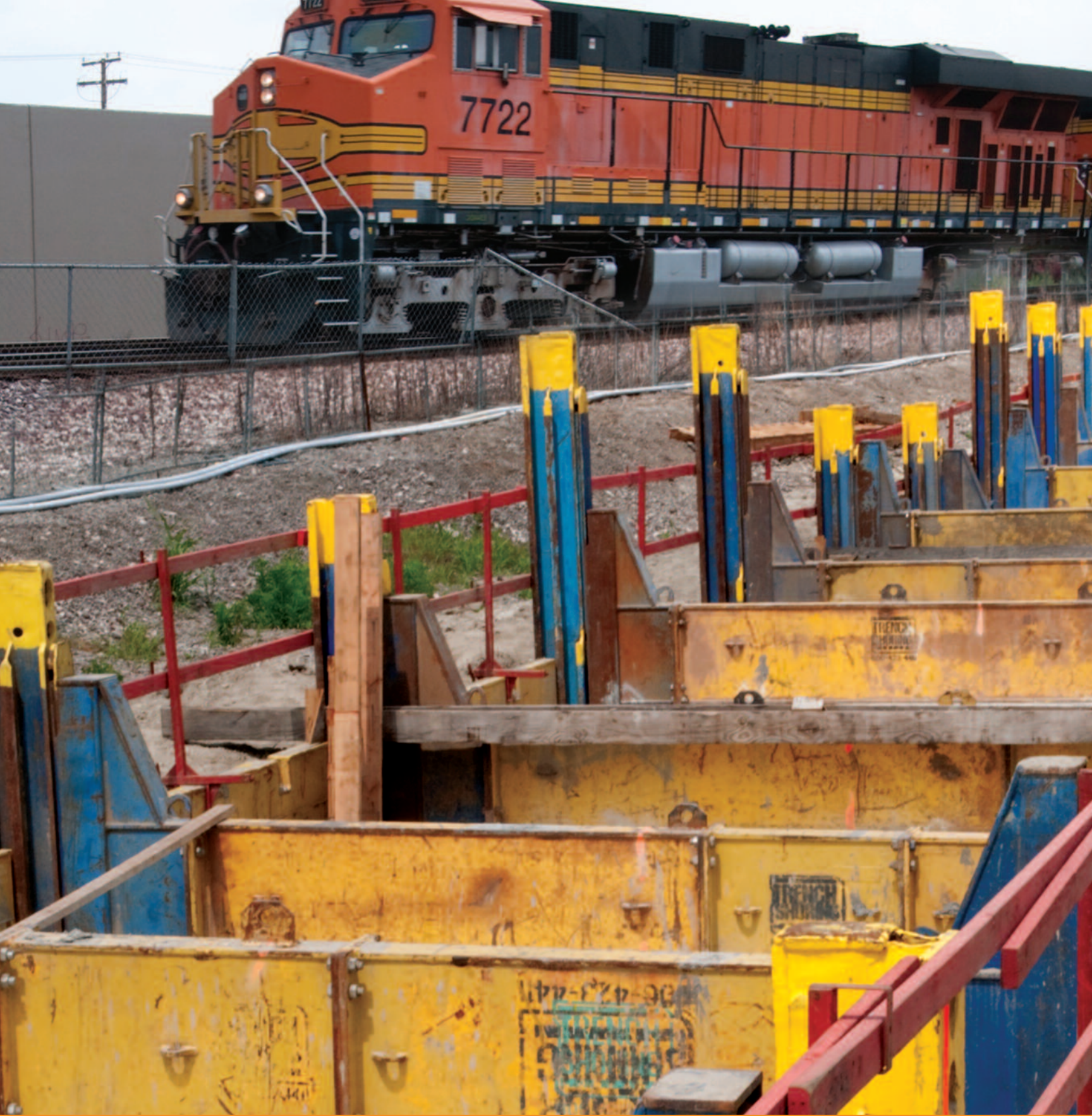
Slide Rail 4-Sided Pit w/Utility Panels
