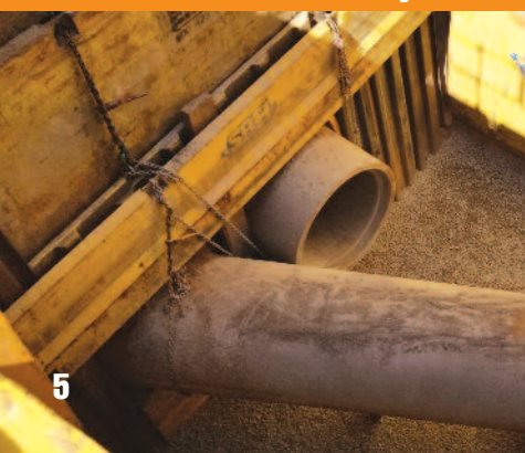
Slide Rail 4-Sided Pit w/Utility Panels
