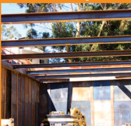
H-Beams & Shoring Plates
