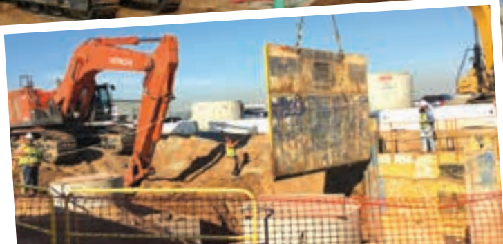
Top Left: Granite Construction uses a Komatsu 490 excavator rented from Savala Equipment Rentals to place slide rail in the 24' sewer trench at phase 1 of the MSC North project at LAX.
