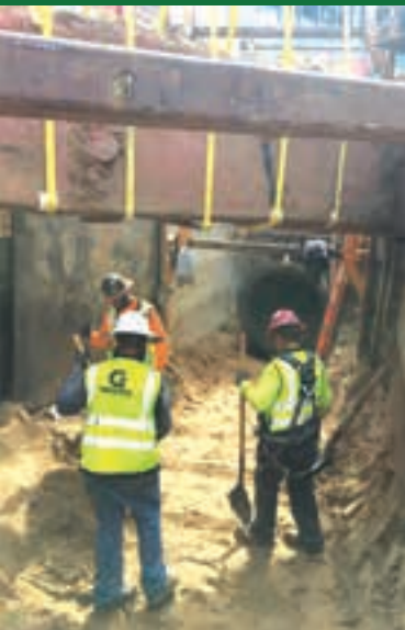
Above: Granite team members working on the 48" storm drain under existing utilities.
