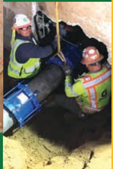
Below: Placing tie-in to bypass existing domestic water.
