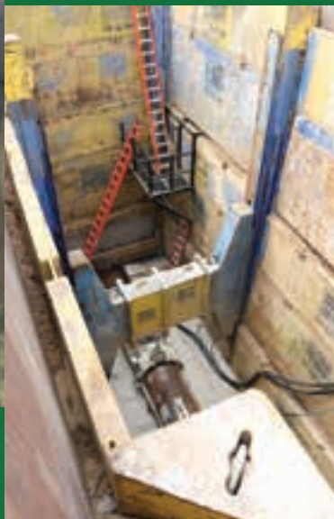
Above: Granite team members working on the 48" storm drain under existing utilities.
