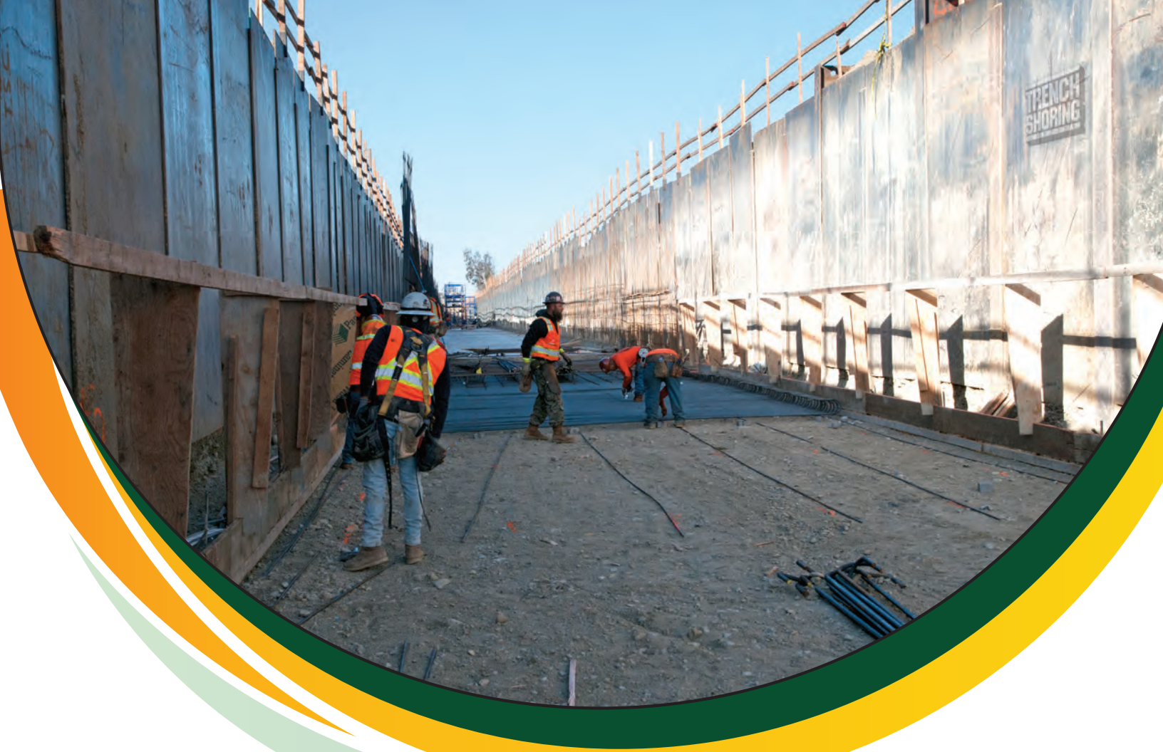
••• • Above: Pacific Steel Group • (PSG) places 25,000 • pounds of rebar a day. •
