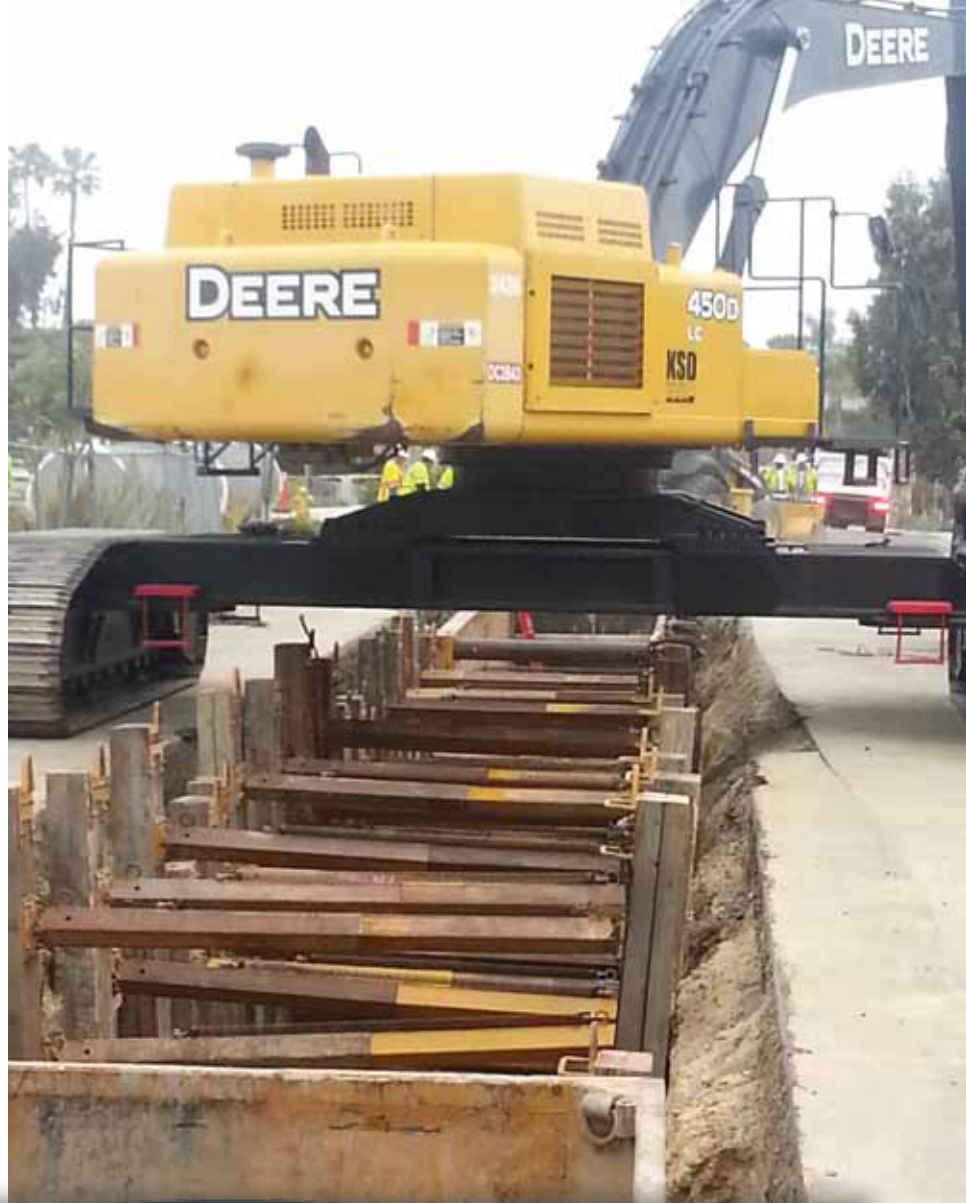
Above: Trench Shoring Company provided the Trench Shields pictured here in a section of the 10-mile water delivery pipeline for the Carlsbad Desalination Project.
