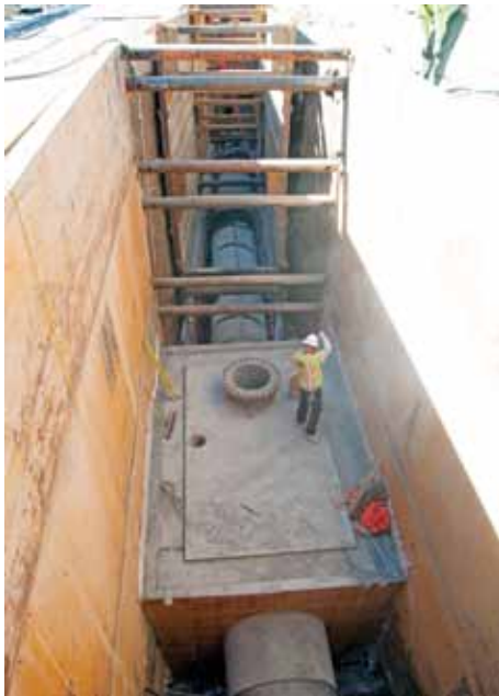
Above: Trench Shoring Company provided the Trench Shields pictured here in a section of the 10-mile water delivery pipeline for the Carlsbad Desalination Project.
