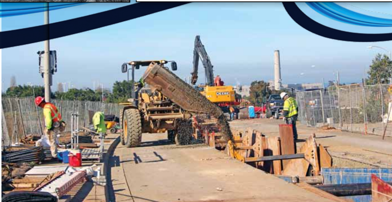
Below: John Deere Wheel Loader filling trench with bedding rock.
