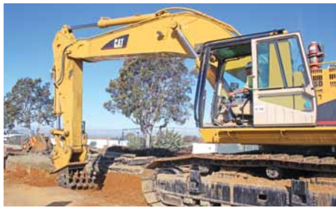
Above: Caterpillar excavator compacts backfilled trench after 52" concrete mortar lined pipe is installed.
