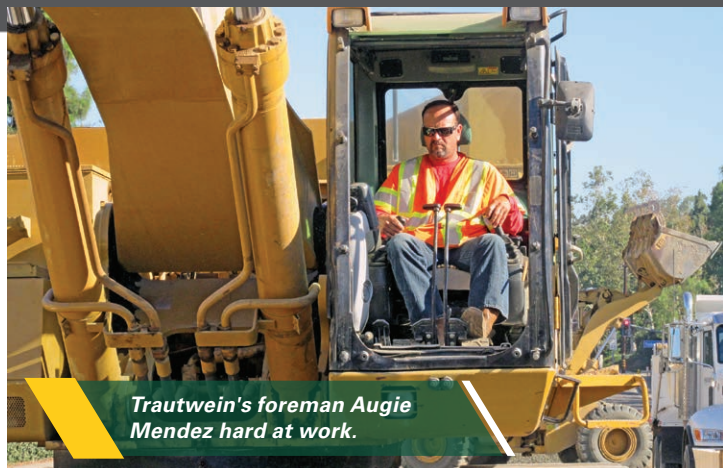
Two Caterpillar excavators backfilling in tandem.
