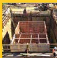
Two bay sheeted pit—re-braced
