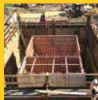
Two bay sheeted pit—re-braced
