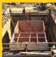
Two bay sheeted pit—re-braced
