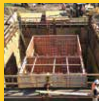
Two bay sheeted pit—re-braced
