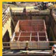
Two bay sheeted pit—re-braced
